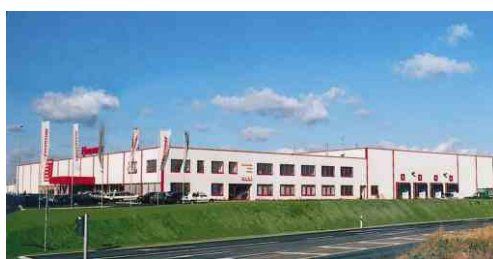
Central Warehouse Ostrau
