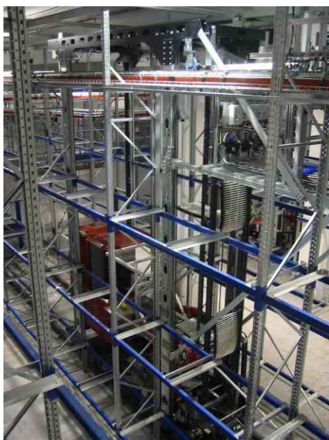
Batch Pick Mobile in the storage bay aisle
