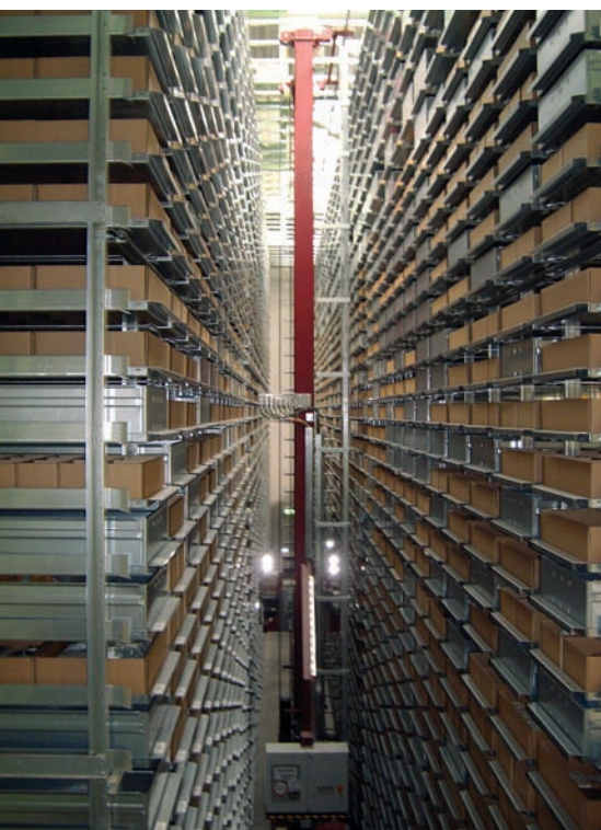
Foto: Westfalia Storage Systems
