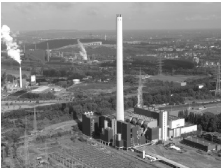
Müllheizkraftwerk in Essen-Karnap, betrieben von der RWE Power AG. Waste-fuelled power plant in Essen-Karnap (Germany) operated by RWE Power AG.
