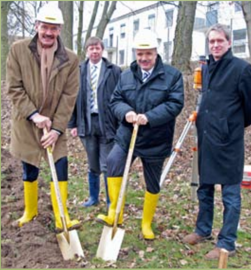
from left: Harrie Swinkels, Rainer Steinbach, Rudolf Keller, Matthias Versbach at the first cut of the spade
